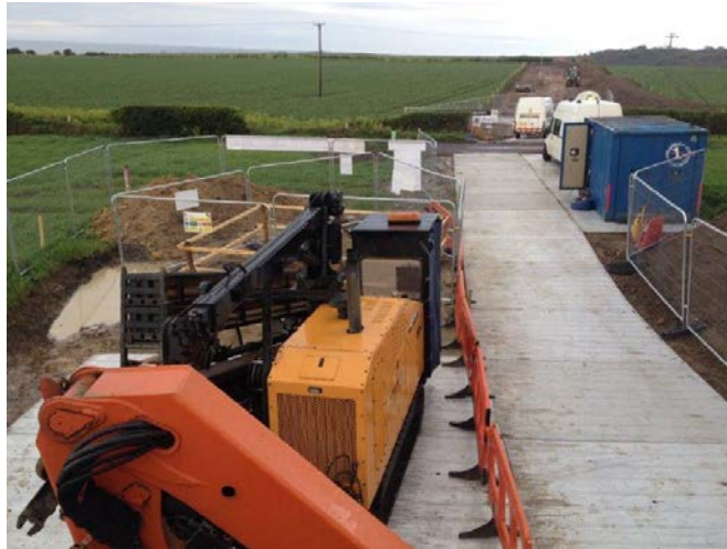
Figure 5 Typical launch pit complete with aluminium track.
